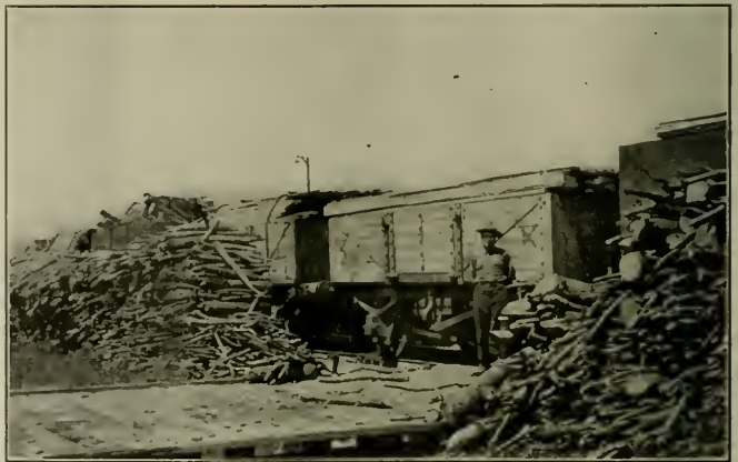
TRAIN IN FUEL YARD IN FRANCE.
